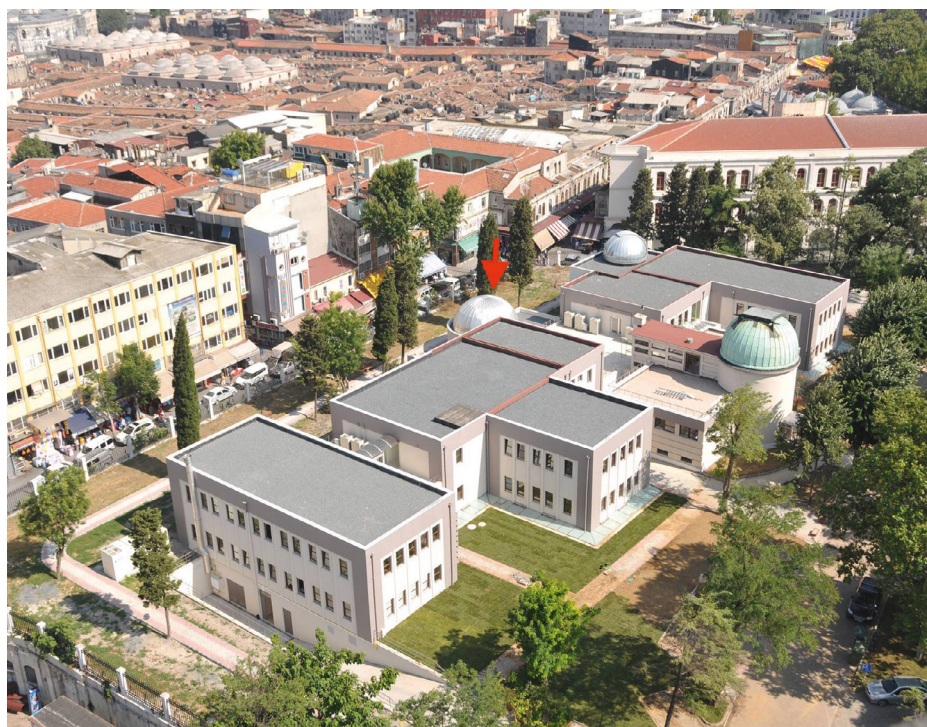
Figure 1: The Department of Astronomy and Space Sciences complex at Istanbul University. The historical and modern domes for telescopes and the planetarium (marked with a red arrow) are noticeable. Image Credit: Istanbul University
