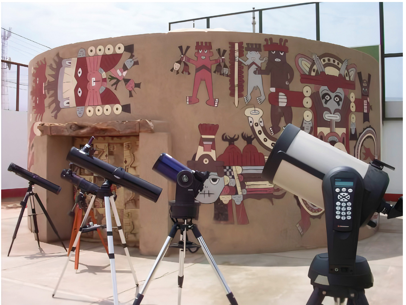
Figure 2: The exterior of the María Reiche Planetarium, built of "adobones" and cane. This image also shows the telescopes used for observation after the performances, weather permitting.
